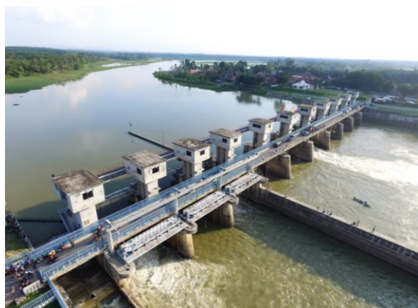
Figure 3 Perjaya Dam in OKUT
