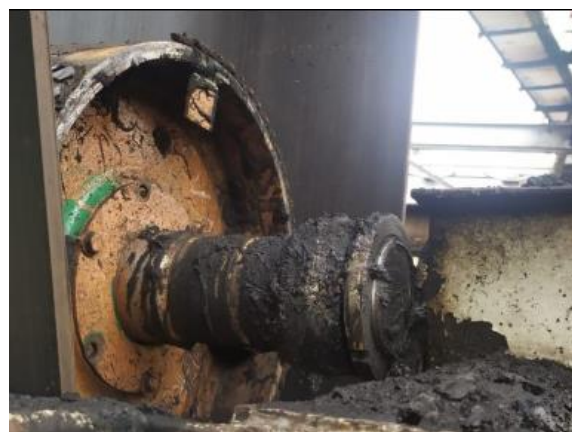
Figure 7 Condition of the pulley shaft on the bearing side.
