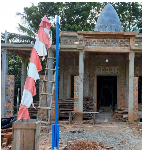
Figure 2 Solar power plant pole installation documentation in Dabuk Rejo village
